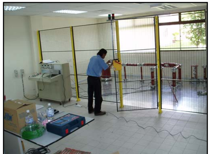
Installation of Safety Net
