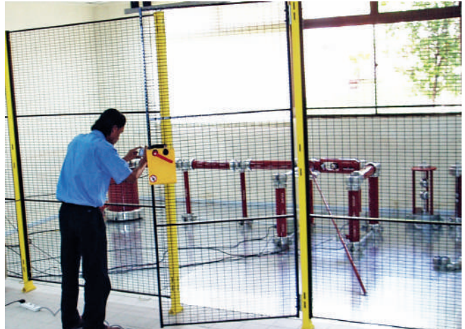
Installation of Safety Fence
