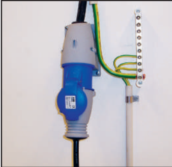
Power Supply for HV9000 is 220/230V, 50/60Hz single phase. Fuse 25A D characteristic.
